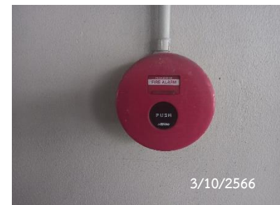
Fire Alarm Manual Station
